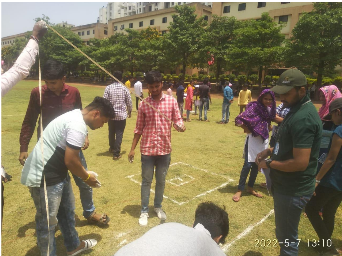
A field training for lining out of building
