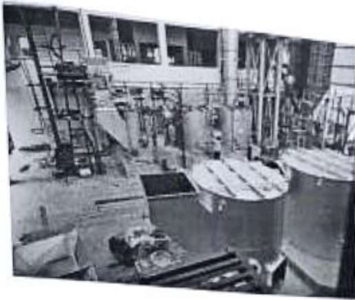
Hazardous Waste Plant
