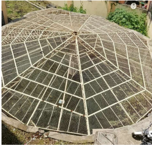
Open well in campus
