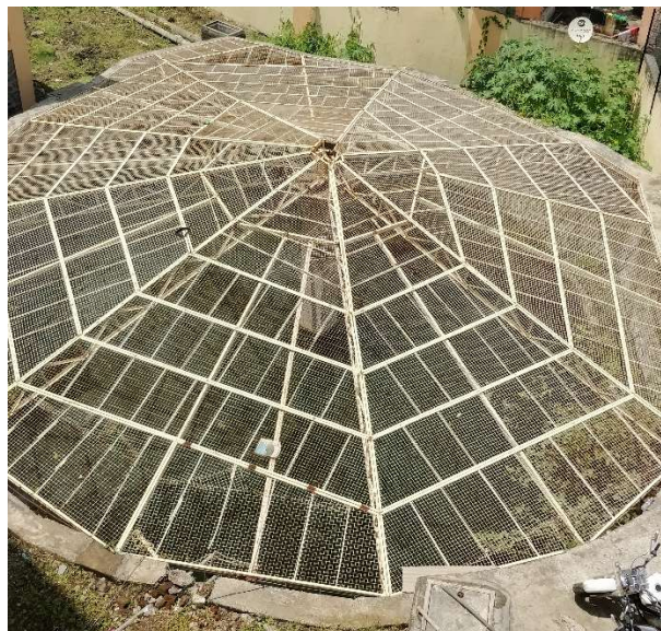
Open well in campus
