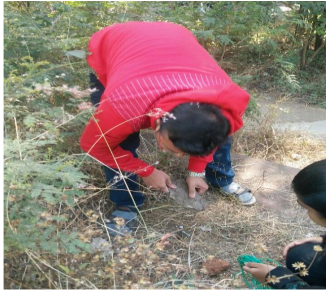
Measuring Earthing Parameters
